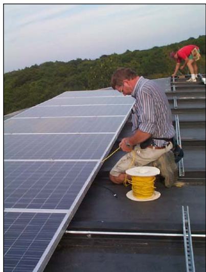
We have installed an array of 88 ASE Photovoltaic panels at the Gilman Ordway Campus.
